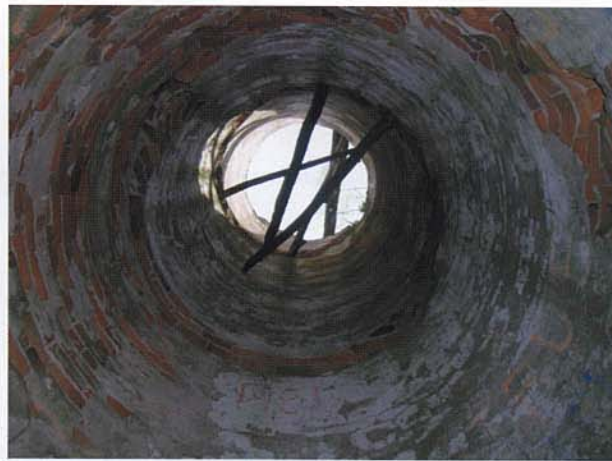
View from inside the tower.
