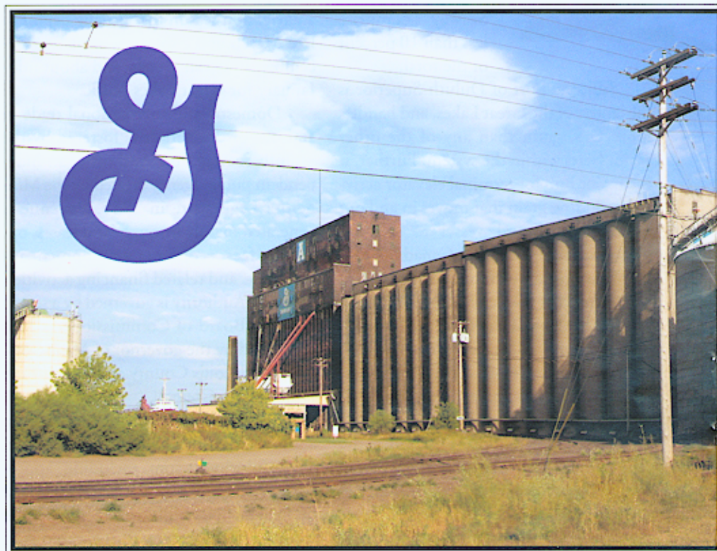
Elevator A was built in 1908. Its steel tanks were added in 1977 and the Port Authority-financed
