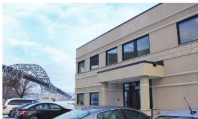
In 2010, AMI Consulting Engineers P.A. moved its corporate office location from Duluth to 91 Main St. in Superior. AMI also has a branch office in Virginia, Minn.
