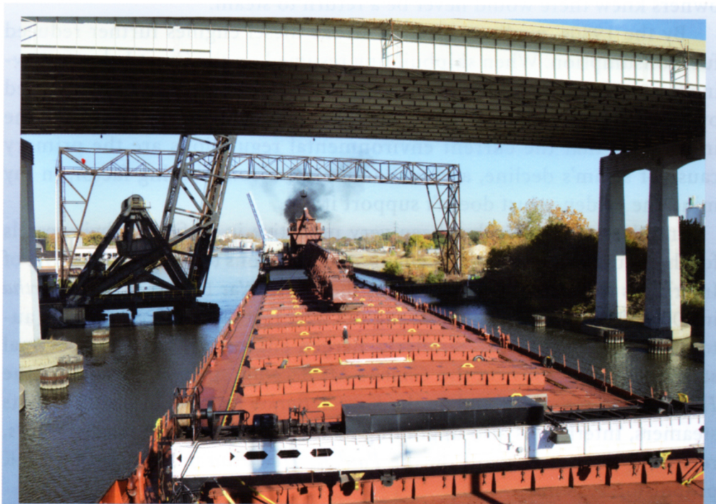
The Jackson winds its way slowly out of the Rouge River, passing beneath I-75. In the background is ca. 1921 Norfolk-Southern Railroad bascule bridge. The raised span of Fort Street bascule bridge is in the distance.
