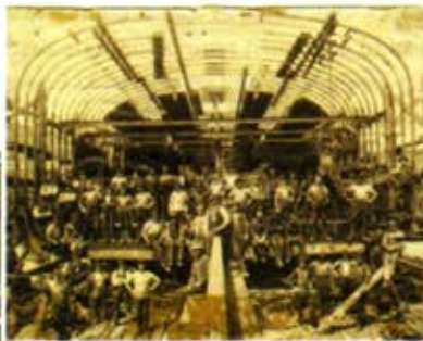
Laborers in whaleback under construction, Duluth, Minnesota.
